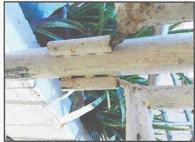
ACTUAL PHOTOS OF TENT FRAME SLOTS AND TRUSSES
